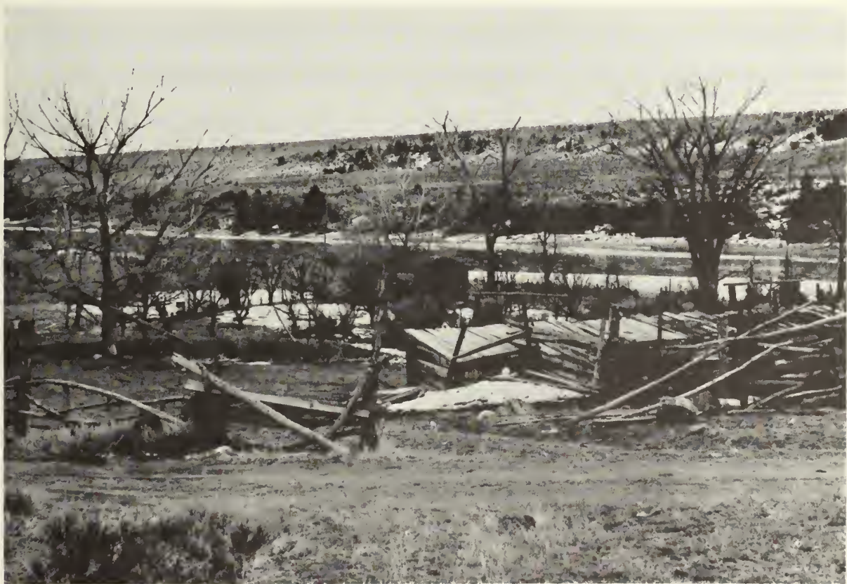
Photo 40. Corral, sheds, stone house, and addition in 1962. (Photo Credit: Utah State Historical Society).
